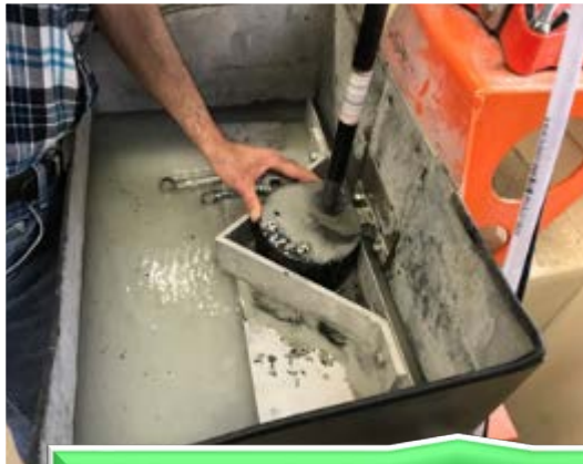
4. Coring the holding holes
