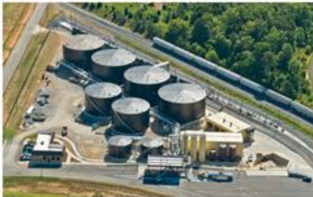
SAMPLE 'A' ASPHALT CEMENT SUPPLIER'S TERMINAL
