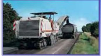
Asphalt Pavement Removal
