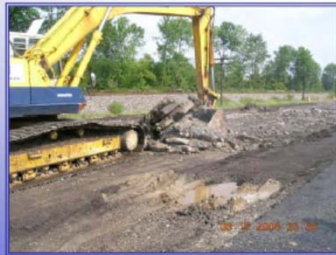
Asphalt Pavement Removal
