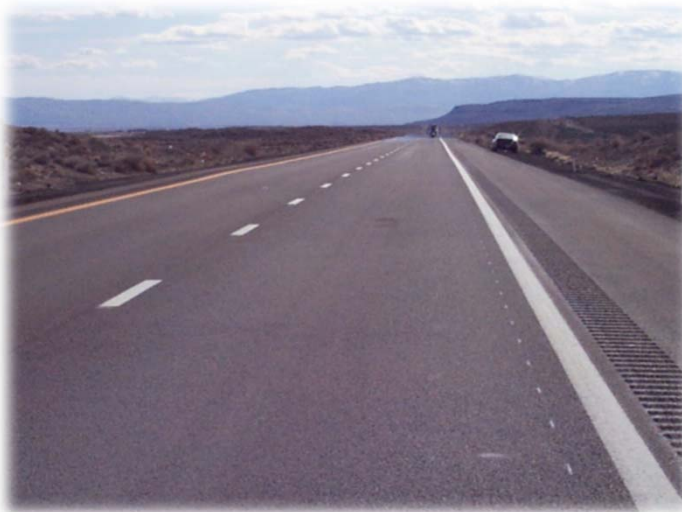
PG 64-22 modified, no rutting
