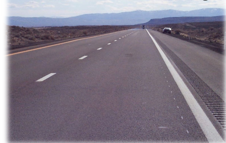
PG 64-22 modified, no rutting
