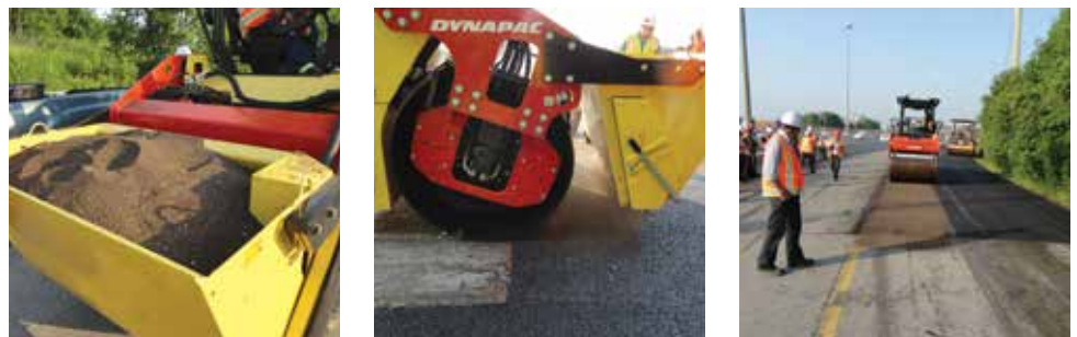
Figure 2 SMA Pavement – Gritting Sand Application
