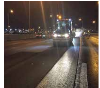
Figure 4 Placing and Rolling SMA Mix
