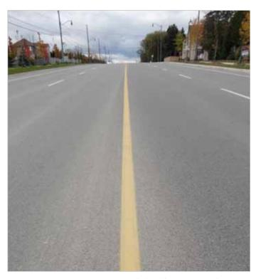
Properly constructed cold joint five years after paving.
