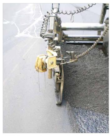
End gate all the way down and proper overlap.
