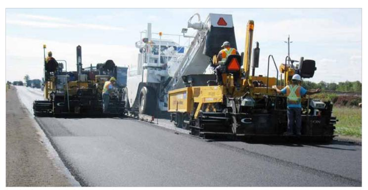
Paving in echelon with warm mix asphalt on an MTO project.
