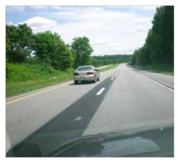
Patching of the longitudinal joint extends pavement life.
