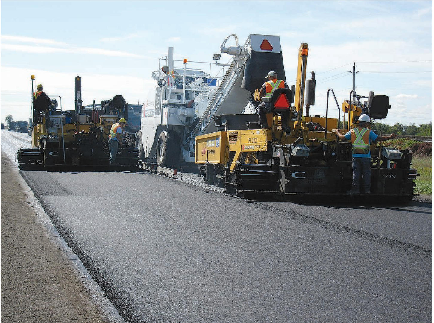
Paving in Echelon with WMA.
